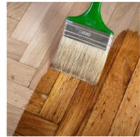
Polyurethane varnish is highly durable. Oil-based polyurethane is a highly durable finish, but it is also easy to apply. It is resistant to heat, chemicals, and wear and tear such as scratches. When applied according to directions, oil-based polyurethane supplies a lustrous finish that deepens the color of the wood. Water-based polyurethane will not penetrate the wood as deeply, and also does not add color to the wood.
