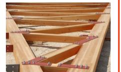
Laminated timber is also used in the construction industry. By laminating a number of small pieces of timber together into a single large beam it is given greater strength to resist the forces that create bending, compressive and tensile loads in structures.
